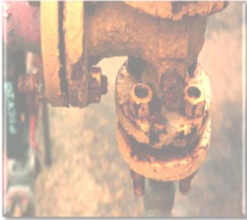
Insufficient bolts
