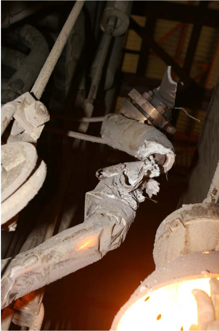
Tube 161 lifted approximately 16 ft (view looking up)
