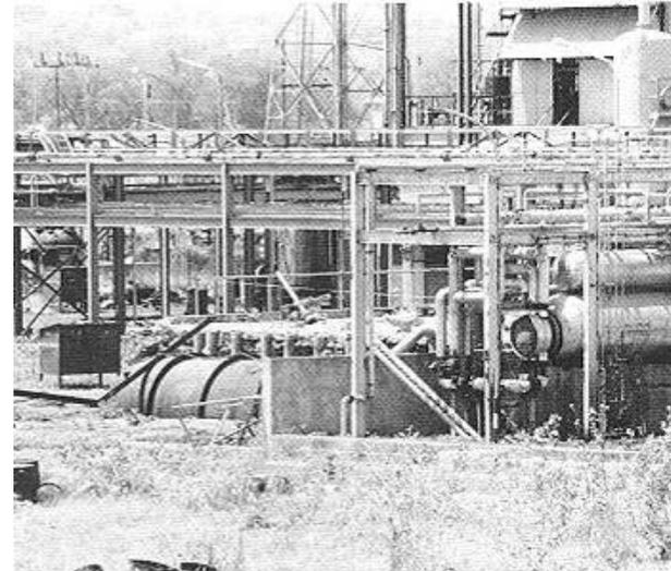
Water entered tank 610 in foreground of picture reacting with MIC and caused an uncontrolled release of a vapor cloud.
